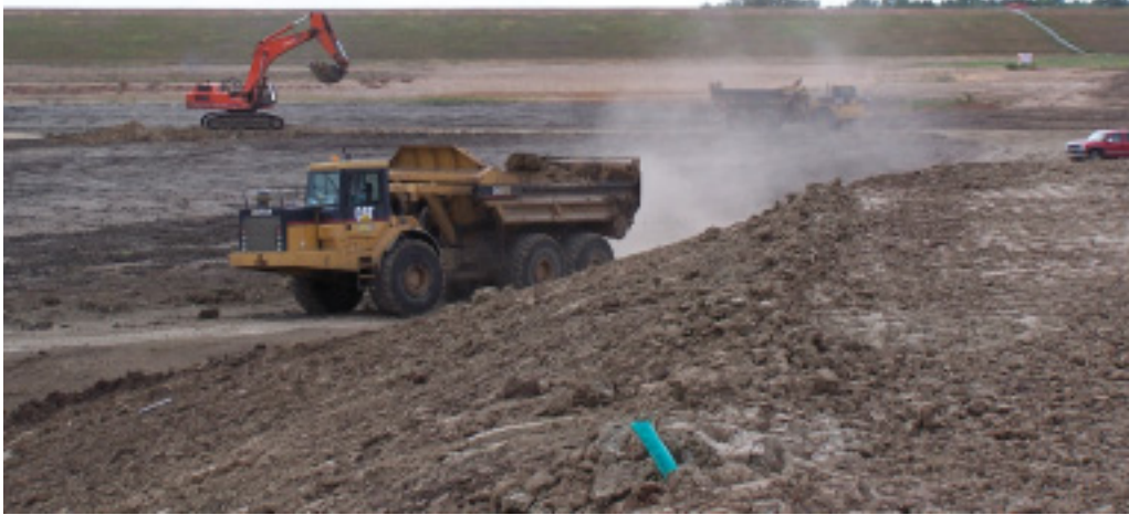
Figure 3.6: Removing sediment from a flood-control lake. A dam is in the background.
