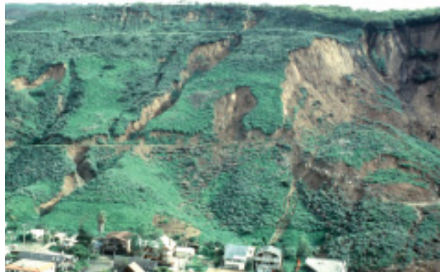
Figure 6.6: 1994 landslide (USGS photo).
