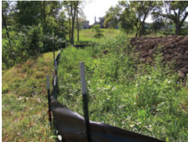
Figure 3.10: Silt fences collect sediment and keep it from reaching water bodies near construction sites. Construction is just starting on this site.
