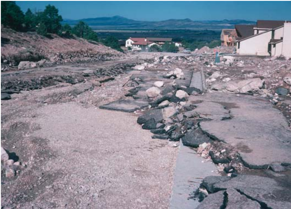
Rocks and debris litter a roadway after a flash flood in Weber City, Utah. (NRCS photo.)
