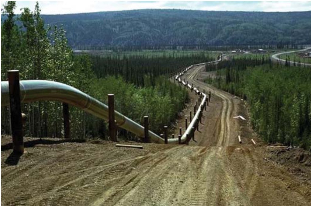
Permafrost-affected soils with loamy textures become saturated and unstable if allowed to thaw. In areas of these soils, the trans-Alaska oil pipeline is elevated above the ground. (Photo by Alaska NRCS staff.)
