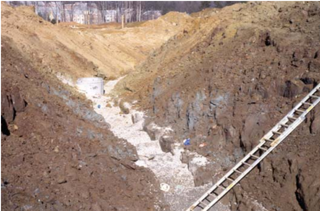
An adequately sloped trench.
