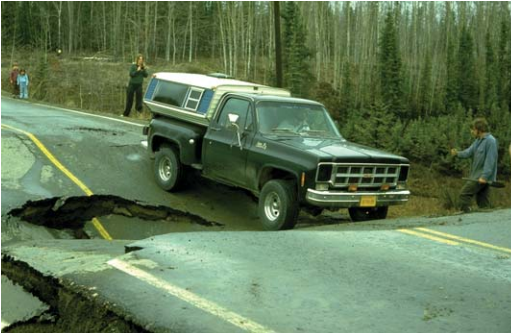
Collapse of a section of the Alaska Highway in 1982 after massive ice under the roadbed melted. (Photo by Joe Moore, USDA, NRCS).
