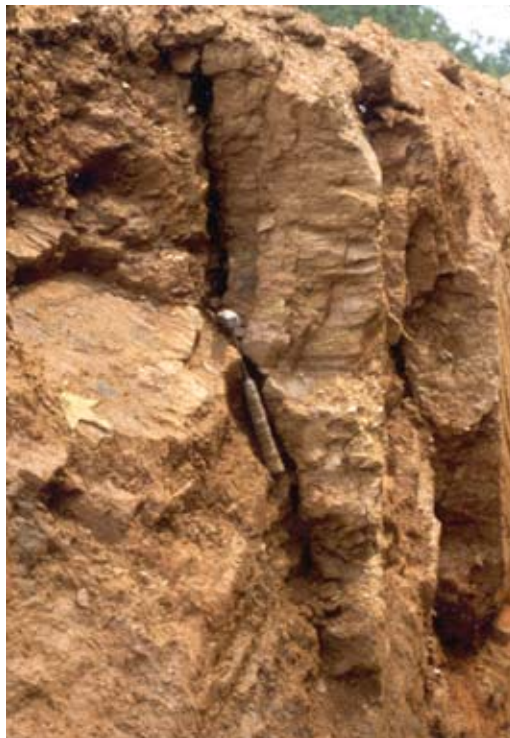
Fissures developed in a trench wall along natural zones of weakness in the soil profile. Note hand pick for scale.
